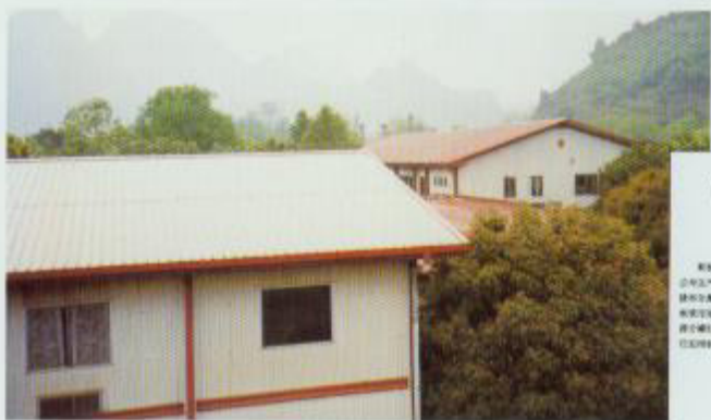
• 桂林甲山饭店 - 采用彩色镀铝锌钢板的来实屋，墙面板使用 18 年后仍处完好状态 Gullin Jiashan Hotel - LYSAGHT® profiles produced from Colorbond® steel after 18 years are still in excellent condition.
