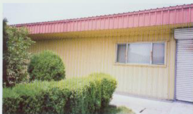
• 奉堂岛华基邦道制管厂 - 紧靠海边，采用彩色镀铝锌钢板的来实屋，墙面板使用 13 年后仍处良好状态 Huayan Bundy Tubing - After 13 years by sea, LYSAGHT® profiles produced from Colorbond® steel after 13 years are still in good condition.
